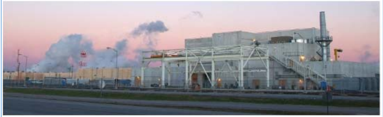
Figure 8-7. The depleted uranium hexafluoride (DUF6) Conversion Facility at the PGDP.
