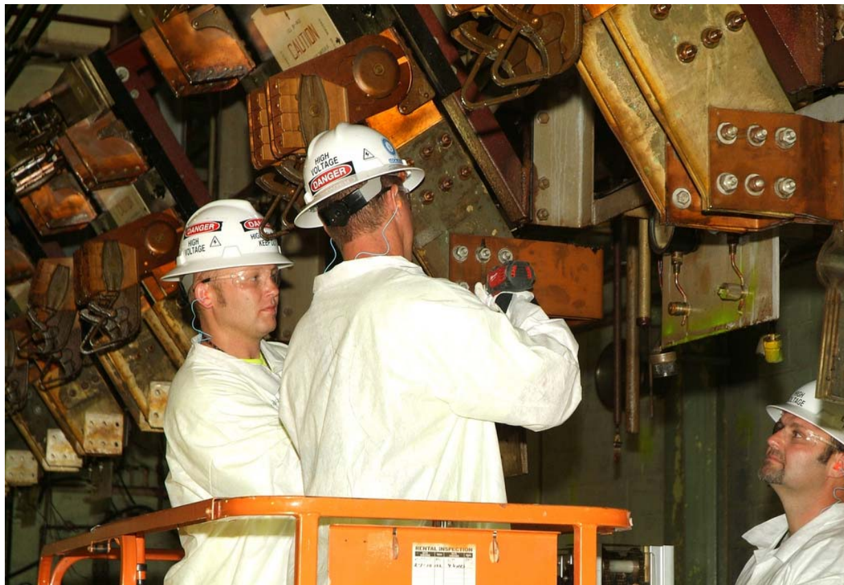
Figure 8-1. Maintenance and decommissioning work on electrical systems at the PGDP.
