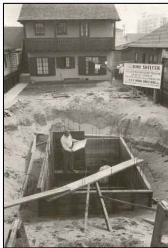
Figure 6-7. Home fallout (bomb) shelters under construction in the 1950's.
