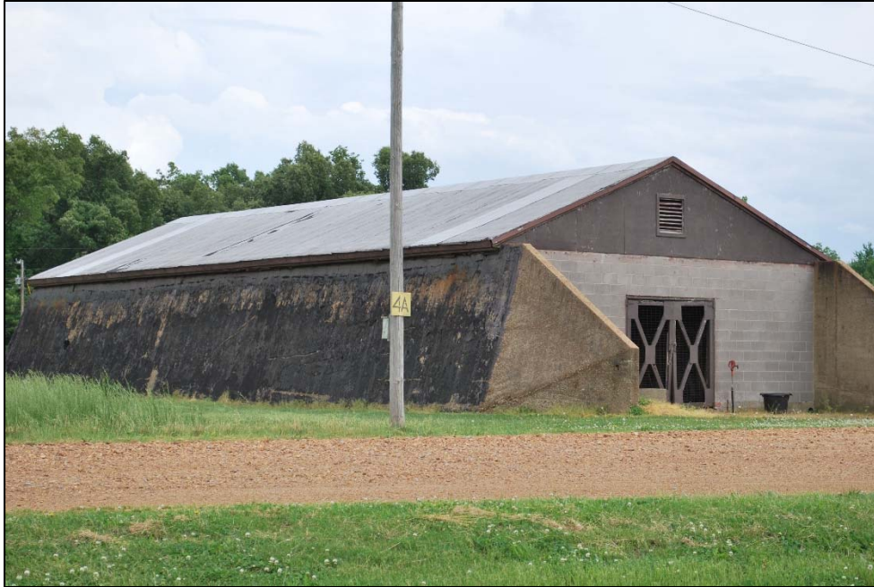
Figure 6-6. Abandoned KOW TNT storage bunkers on the DOE PGDP Reservation
