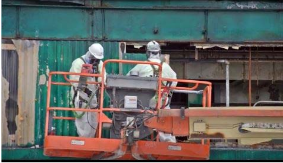
Figure 8-12. C-410 demolition workers in personal protective gear.
