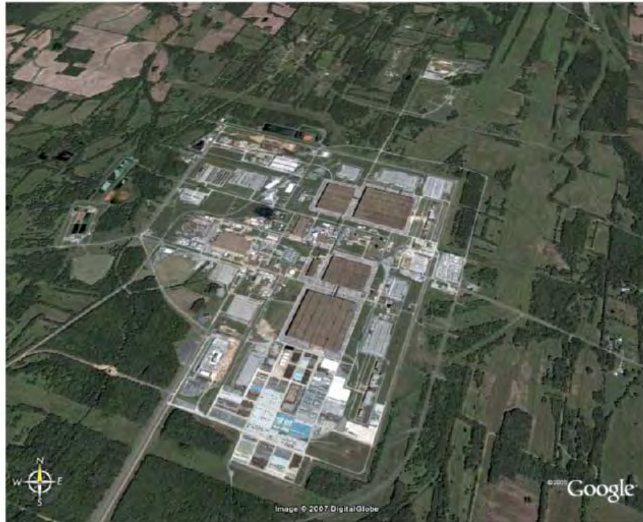
Paducah Gaseous Diffusion Plant (PGDP) Paducah KY
