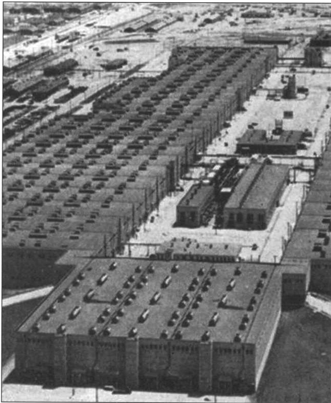
K-25 Gaseous Diffusion Plant at Oak Ridge, Tennessee, was the prototype for the PGDP.
