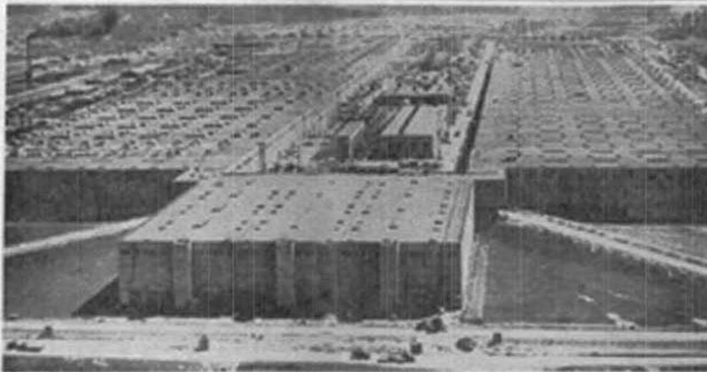
IT IS PRESUMED THAT Paducah's atomic bomb plant will look something like the big factory at Oak Ridge, "home of the atomic bomb." The building planned here may be K-25, the larger gaseous diffusion plant at Oak Ridge. The sides of H-shaped K-25 are 2,400 feet long.
