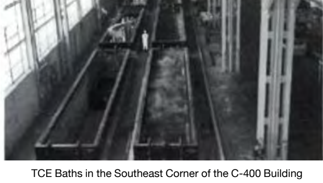
TCE Baths in the Southeast Corner of the C-400 Building
